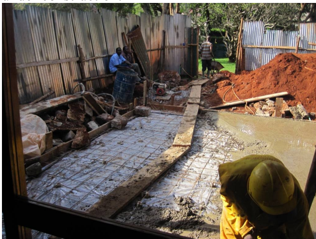
Construction site at MGH
